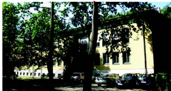
A43: AWI building Seminar Room Offices Stable Isotope Laboratory (Cellar)
